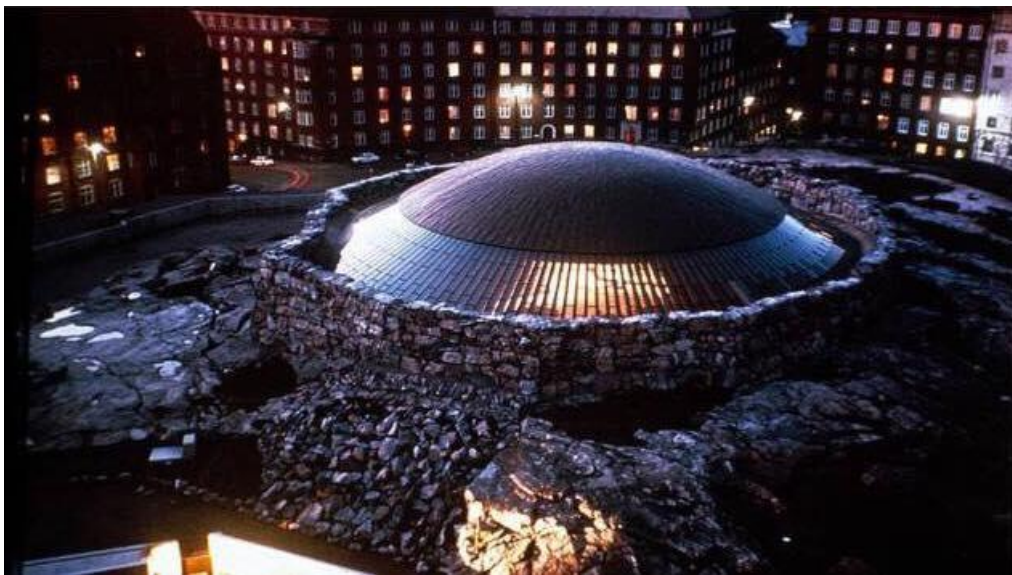
Figure 4: Helsinki Rock Church (Project U 2015)
