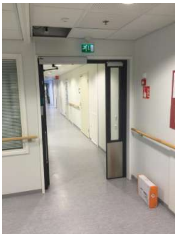
Figure 19: Doors leading from the group home dining and living room area in Villa Toukola.
