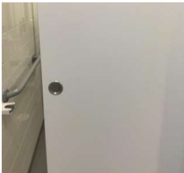
Figure 17: Individual room bathroom door in Villa Toukola
