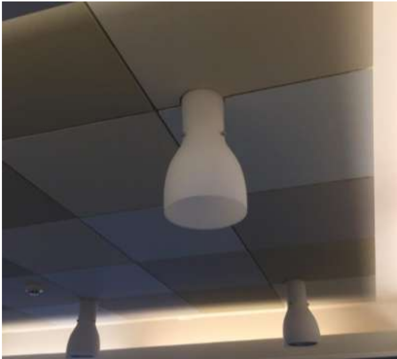
Figure 20: Noise cancelling material used in the group home's dining area of Villa Toukola
