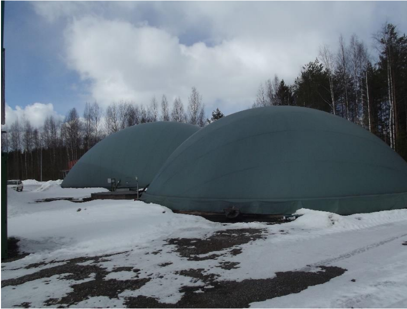
FIGURE 5 Biogas reactors (750 m 3 and 1000 m 3 )
