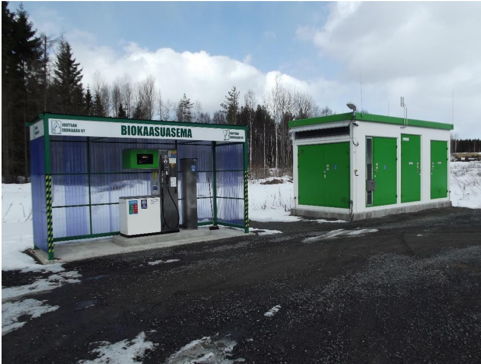
FIGURE 7 Joutsa's biogas plants gas refueling station
