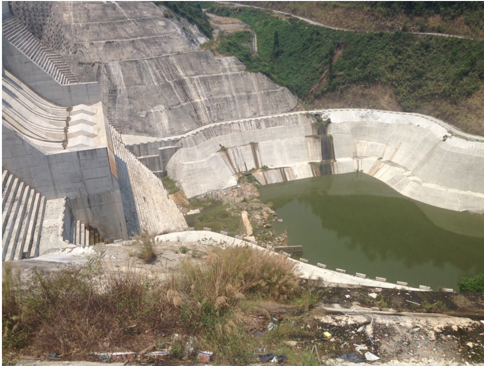
Figure 18: River bed right after the dam
