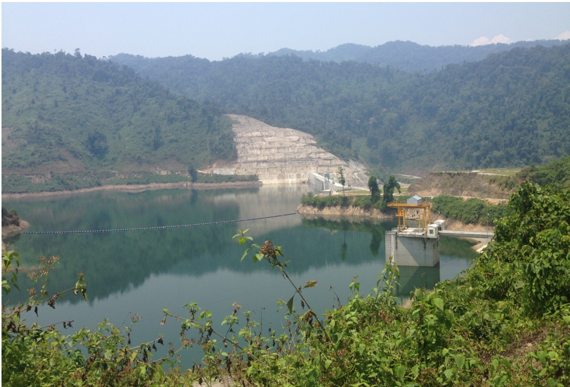
Figure 8: Dam and intake tower
