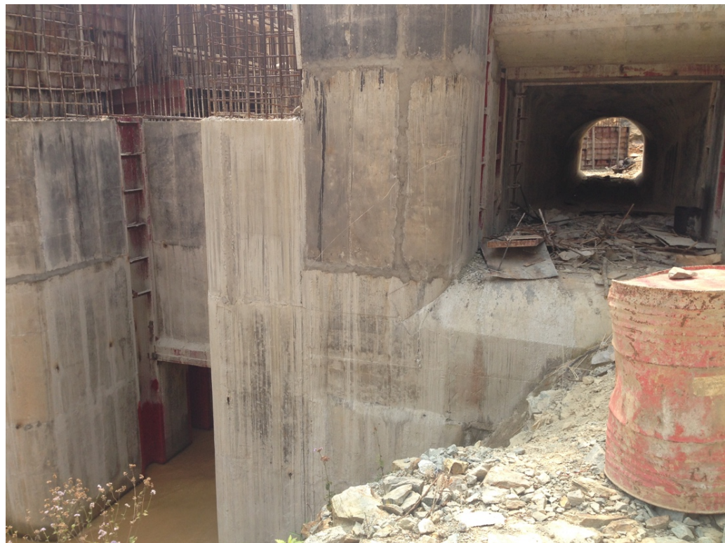
Figure 1: Sediment gate (left) and intake (right) from Nam Pay project
