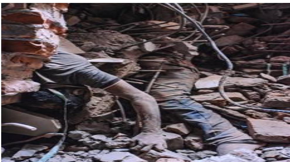
Figure 12: Rana Plaza Collapse (Daily Star 2014)
