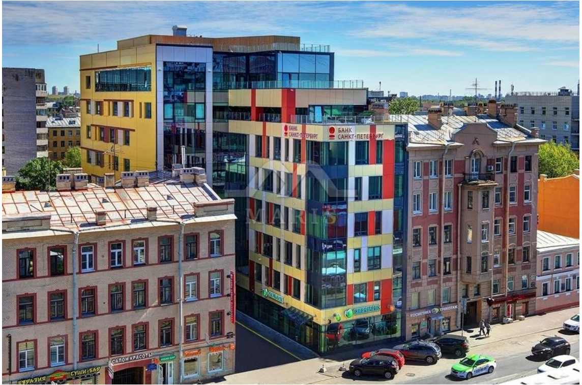
Figure 8. Facade of ECO Status building
