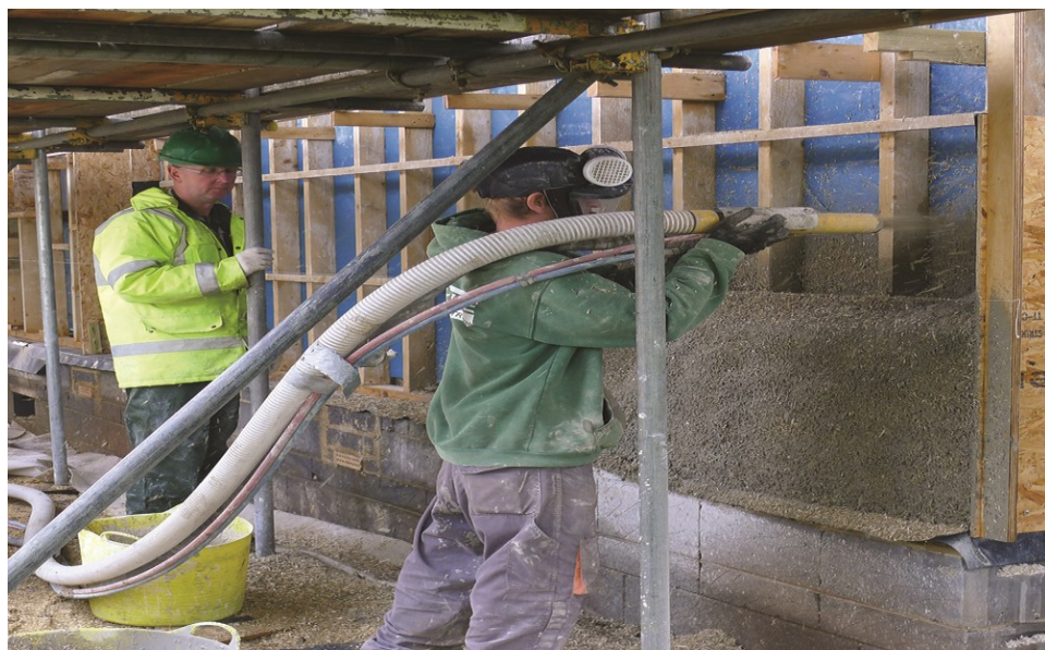
Figure 7 Sprayed Hempcrete on Timber frame (Source: http://www.inmatteria.com )
