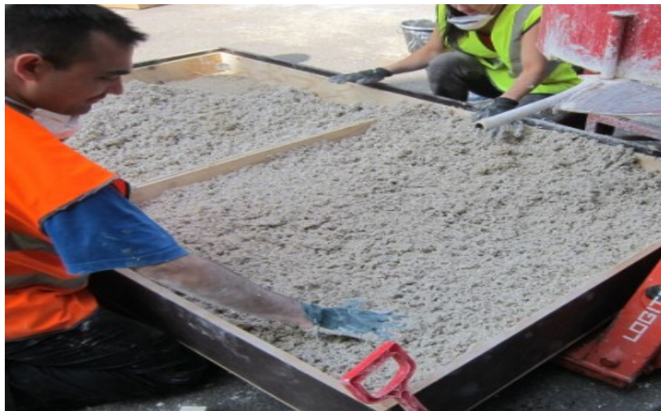
Figure 10 Hempcrete being casted in the test-site by manual tamping
