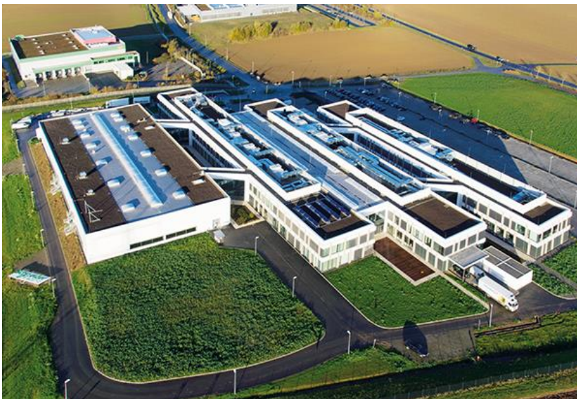
Figure 2. Schneider Electric Automation GmbH Headquarters in Marktheidenfeld. (Schneider Electric [Referred 9.3.2016])
