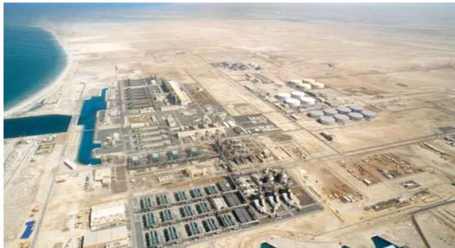
Figure 46 Taweelah A1 Power Plant in Abu Dhabi (United Arab Emirates)
