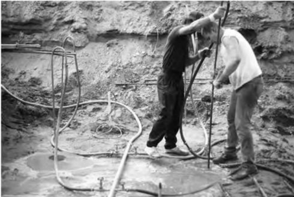
Figure 16. Example of Pre-Thawing Localized Permafrost with Steam Points (Zarling 2015)
