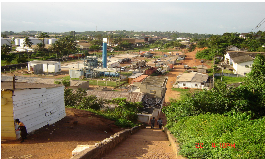
Figure 15 Decommissioning works in Ghana-Benin 19x 12V22 Relocation Project
