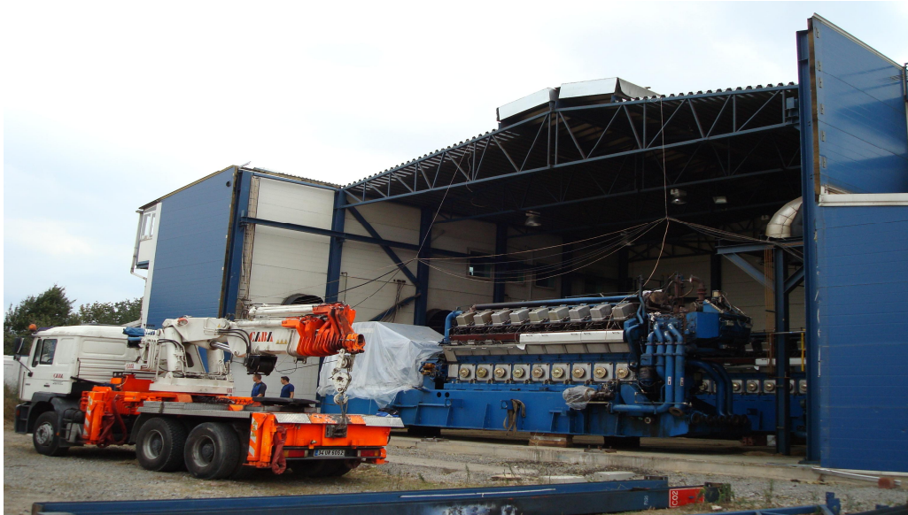
Figure 14 Dismantling power plant in Turkey, Sabodala Mining Company
