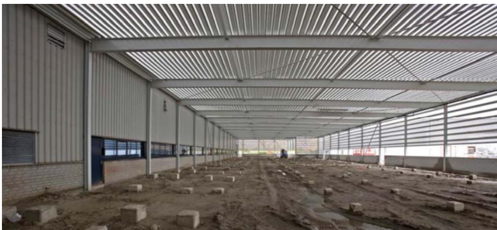
Figure 14. I section beam and column structure example
