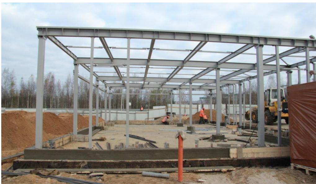
Figure 101. Gas station under construction
