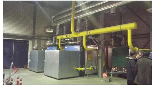
Figure 31: Interior of Test Building
