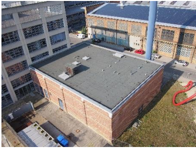
Figure 30: Aerial View of the Test Building
