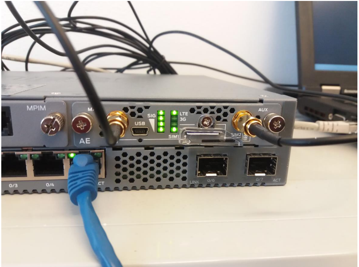
Figure 3. LTE mini-PIM powered on and connected to internet. Both antennas attached.
