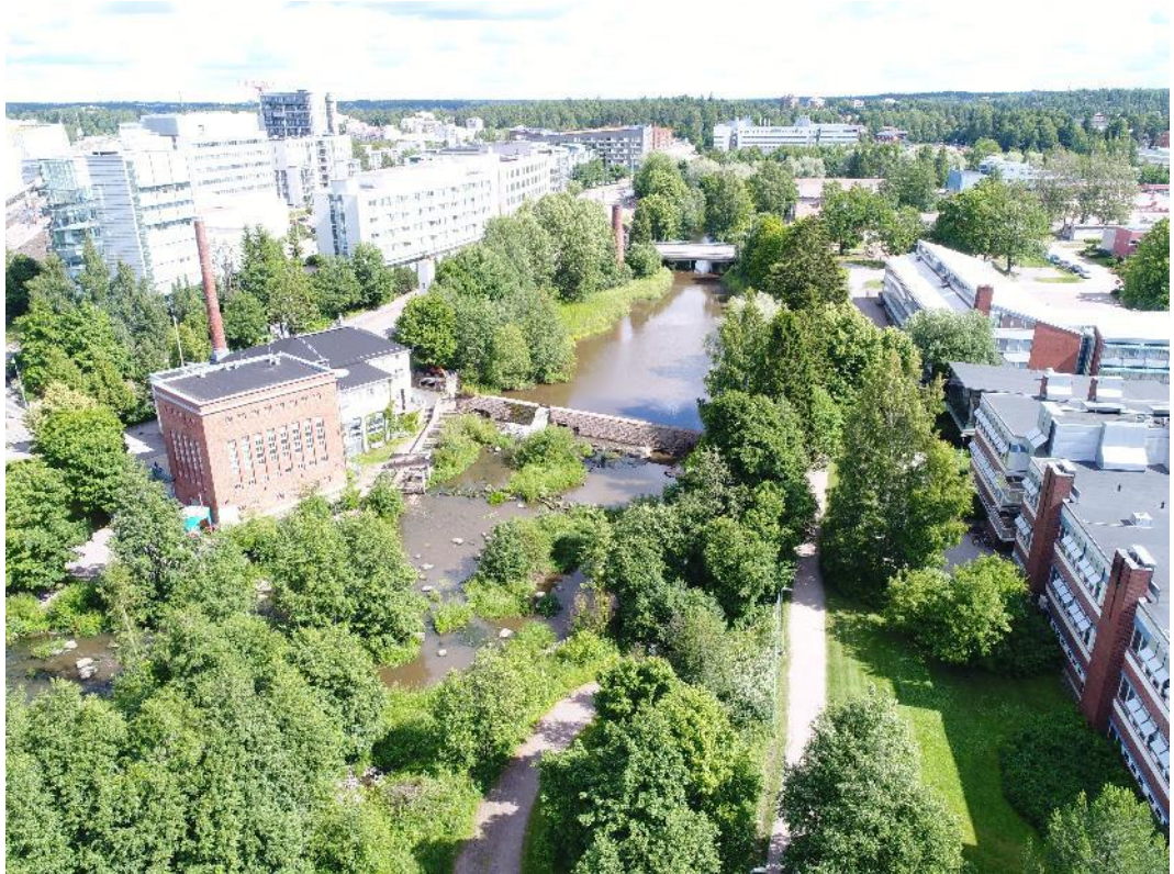
Photo 10. An aerial photograph taken from southwest. In the centre is the dam and next to it on the left side is Vernissa.
