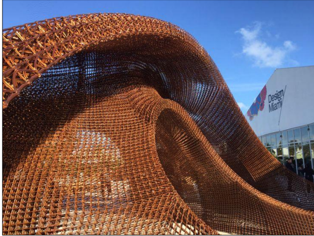
Picture 15. Printed example of architectural structure design by branch Technology Company. Image by: branch technology.
