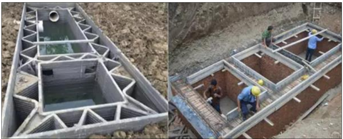
Picture 12. (a) Printed drainage by Winsun™ compare to (b) common way to drainage construction. Images by: 3ders.org, WinSun™ China unveils fully 3D printed public toilets in Suzhou, 2016.
