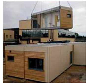
Figure 7. CLT modular unit construction (Pinterest 2016)
