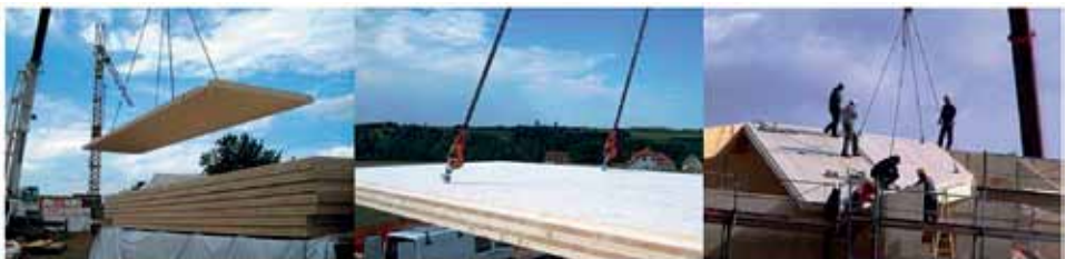
Figure 5. Lifting of intermediate floor and top floor panels (Stora Enso 2013)
