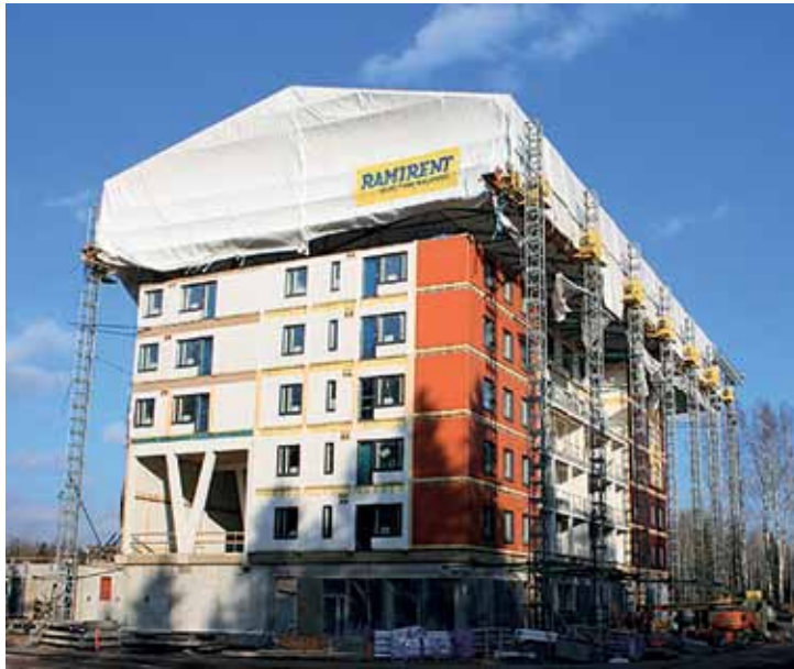
Figure 16. Weather protection (Ramirent Finland Oy 2017)
