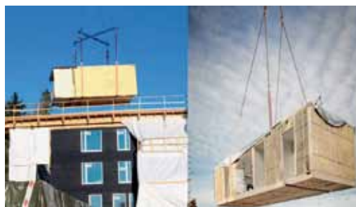
Figure 6. Lifting of modular units (Puuinfo 2017)
