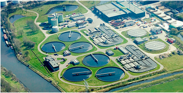
Figure 47. Aerial view of the Amersfoort WWTP (from www.dutchwatersector.com )
