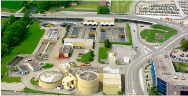
Figure 59. Aerial view of the Kloten WWTP, Switzerland (from www.Poeyr.ch )
