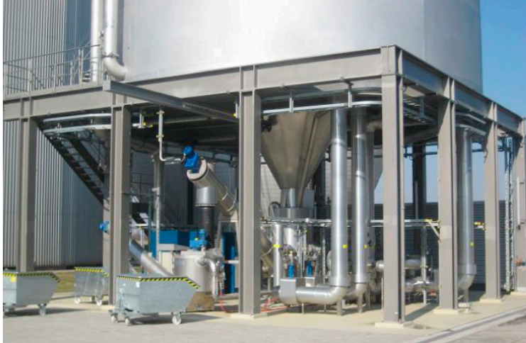
Figure 52. The bottom of the reactor where Struvite is discharged (Nieminen 2010)
