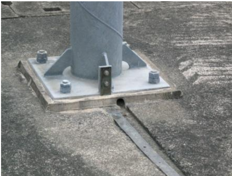
PICTURE 22. Anchor bolt with nut cornerstone (Ahadi 2016, 100)
