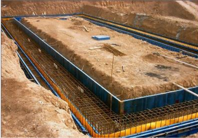
PICTURE 27. Strip foundation in implementation (Fatehipekani & Harischian 2016)
