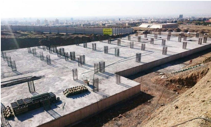
PICTURE 28. Raft foundation in implementation (Mortezaei & Fadavi 2016)
