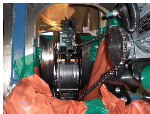
Figure 44. Repair machining ongoing.
