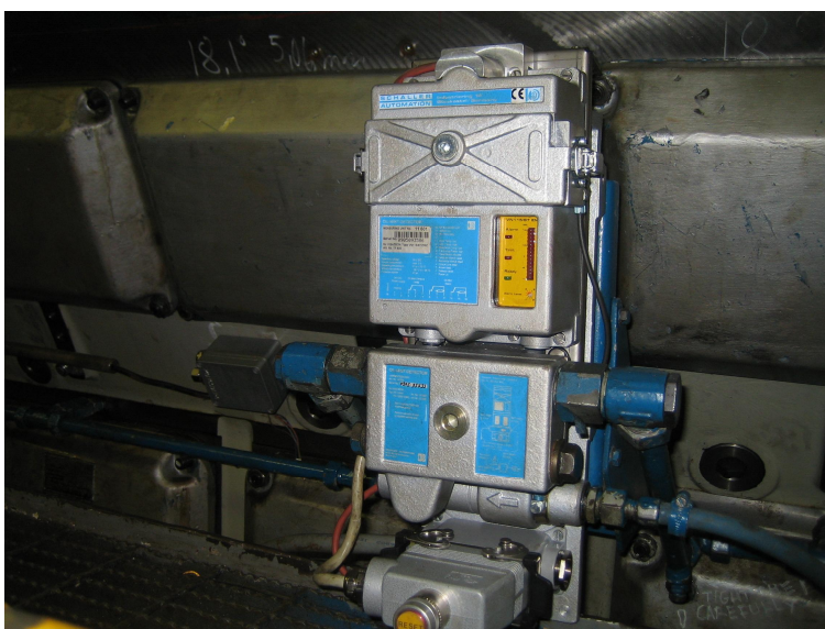
Figure 21. Oil mist detector installed in Wärtsilä Vasa 32 engine. /19/
