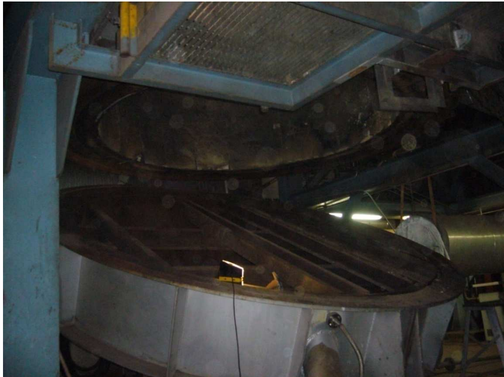
FIGURE 10: Wind chest mechanism opened and grate bearers detached. Primary air duct and fire grate ash disposal visible
