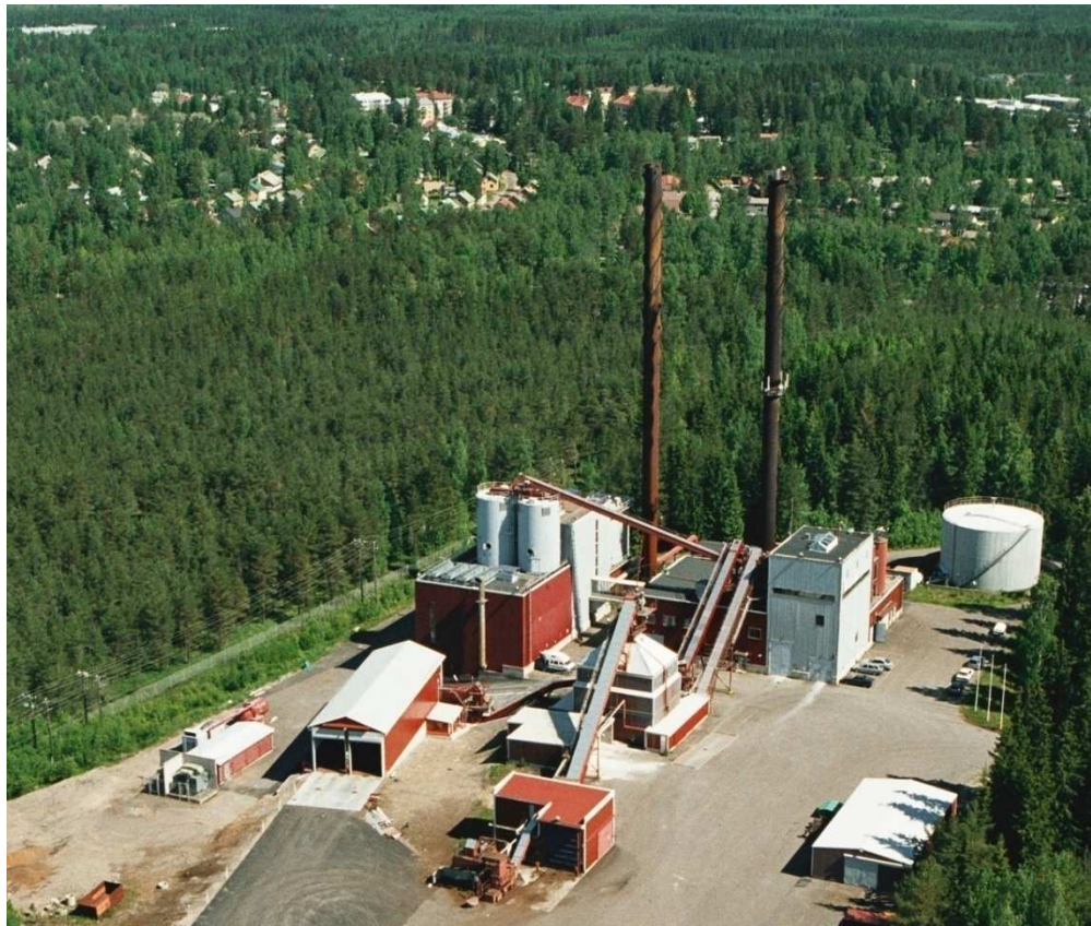
FIGURE 2: An aerial view of Savon Voima Oyj's Pieksämäki power plant. The heat center housing the KPA boiler on the right © Savon Voima Oyj
