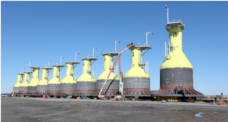
Picture 27: Tahkoluoto foundations in Pori (Offshorewind, 2017).
