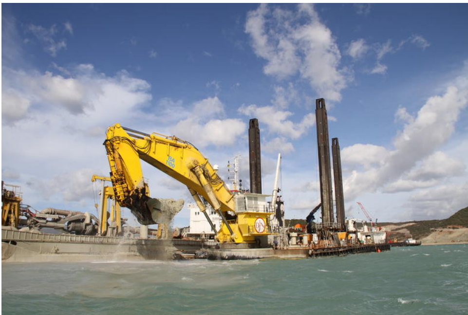
Picture 20: Backhoe dredger Mimar Sinan (JanDeNul, 2018).
