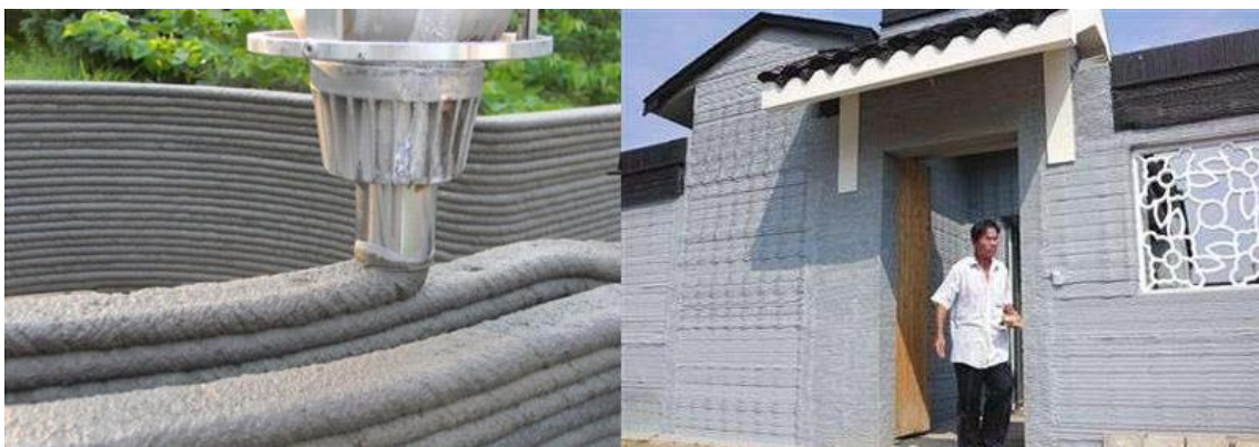
Figure 48. A 3D printed house in Su Zhou in China [71]
