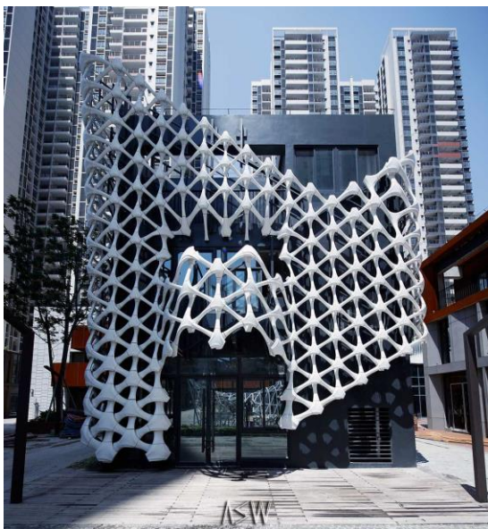
Figure 18. The outer wall Arachne designed and printed by Archi Solution Workshop [30]
