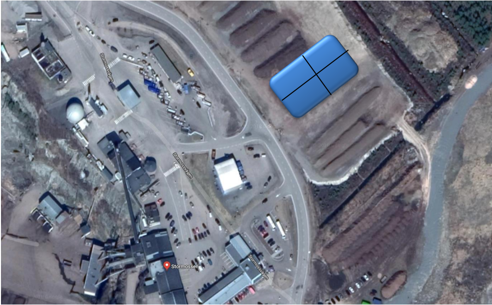
Figure 5. The blue rectangle is demonstrated where the pilot pond will be constructed. [Google Map]
