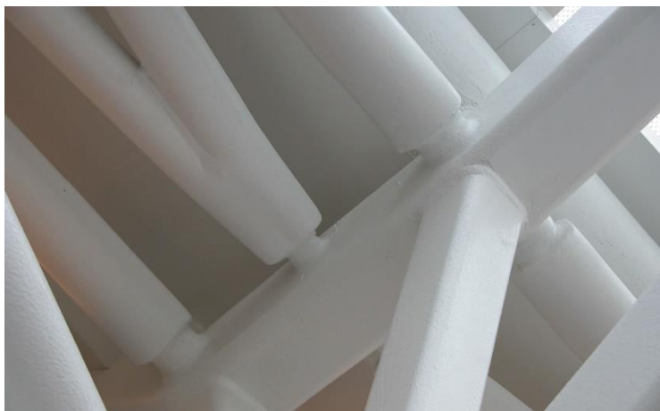
Figure 10. Intumescent coating (5)
