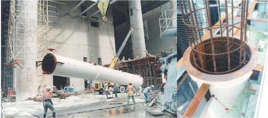
Figure 21. The erection of steel tube column (8)
