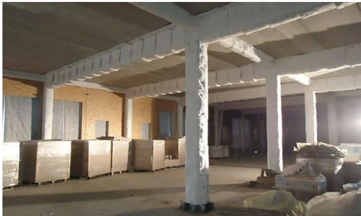
Figure 9. Flexible blanket systems (25)
