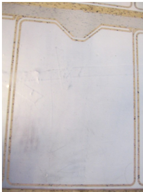
Figure 1. A piece of Elsi floor, photo by Wei Chao
