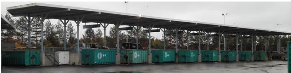
Figure 4. Waste material beds in Kivikko Sortti Station
