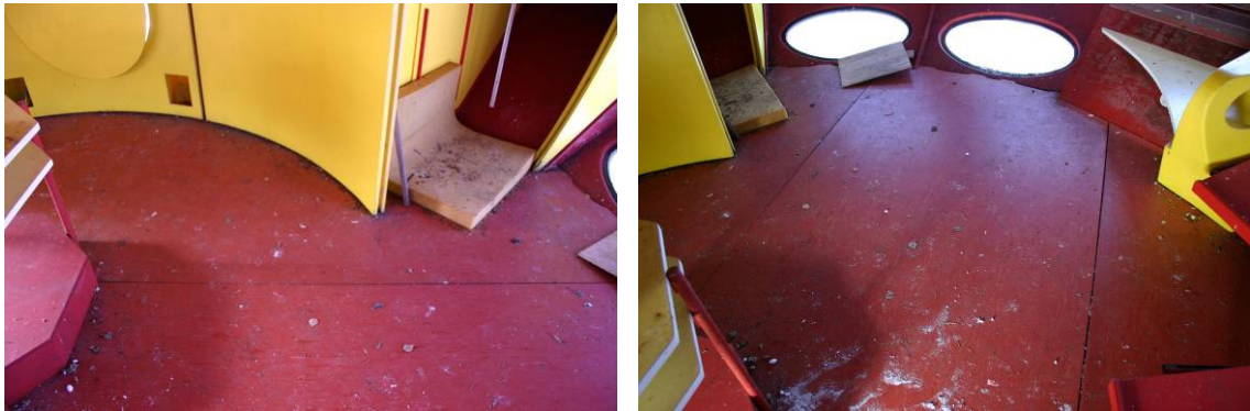
Figure 44. Ventilation holes both side the door. Figure 45. Narrow gaps close to the windows.
