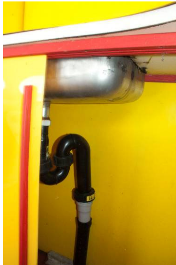
Figure 66. Basin and drainpipe.
