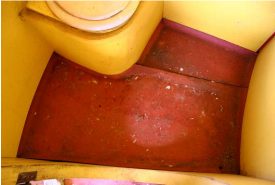
Figure 63. The floor of the toilet.
