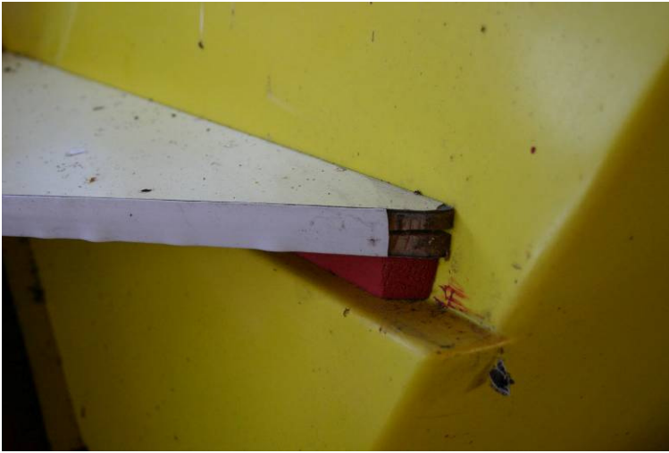
Figure 120. Missing part of the edging strip.
