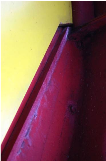
Figure 32. (left) Partition wall set in the mounting batten, which instead is set in the element bent edge.
