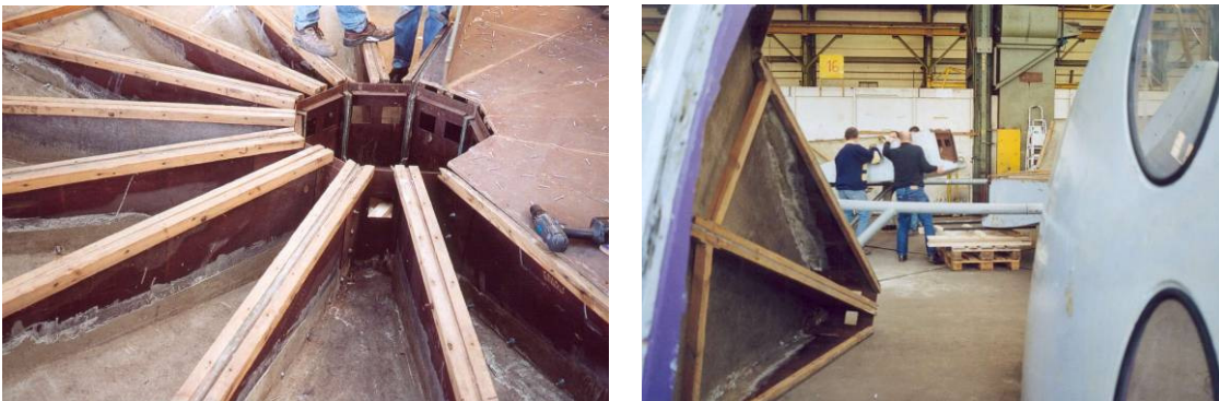
Figure 41. The floor plates are partially dismantled. (Rasier 2002)
