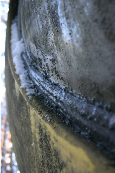
Figure 111. Ice on the window seal. Figure 112. Window seal surface has altered from smooth to uneven. (60-fold magnification)
