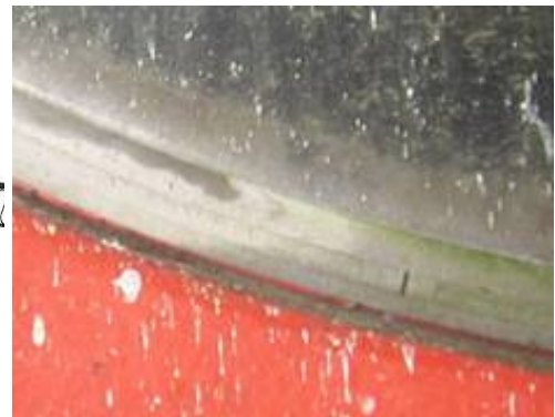
Figure 49. Window seal from inside.
