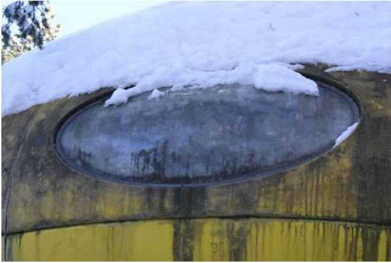
Figure 46. Window from the outside.
