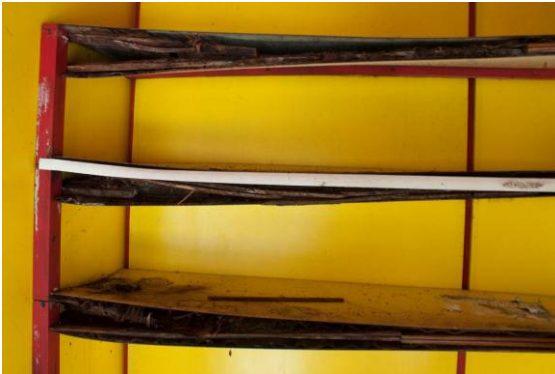
Figure 68. Shelves are made of laminated veneer.
