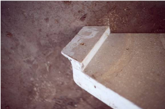
Figure 30. (left) The top of the roof element has a shelter to prevent rainwater from penetrating the structure. (Rasier 2002)
