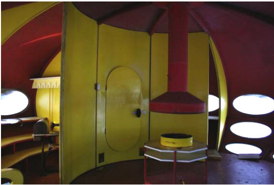
Figure 72. Partition walls are slightly curved.
