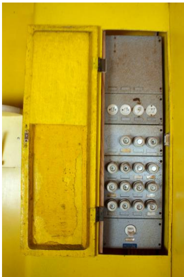
Figure 85. Main circuit breaker in the corner.
