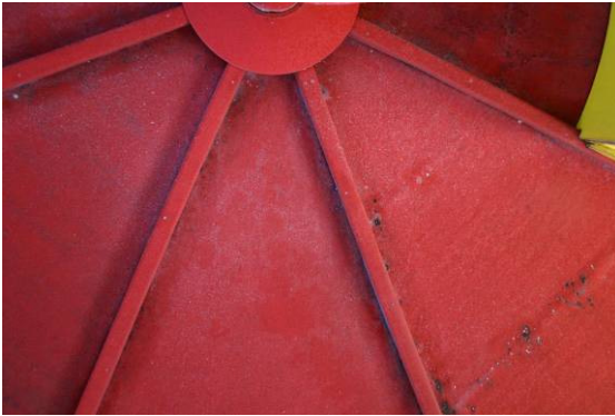
Figure 102. Some elevated areas on the living room ceiling and black deposit.
