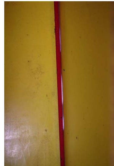
Figure 32. (left) Partition wall set in the mounting batten, which instead is set in the element bent edge.
