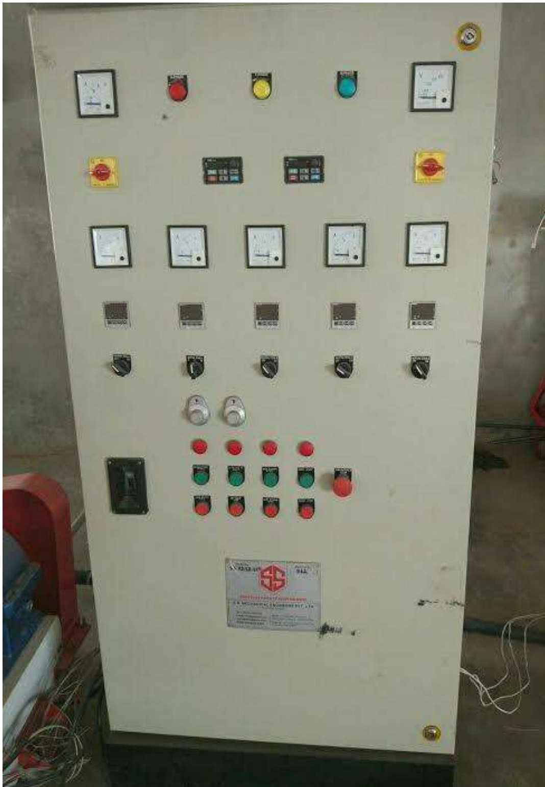
Figure 11. On-off temperature control I at Seti Plastics (Nishan Devkota, 2017)
