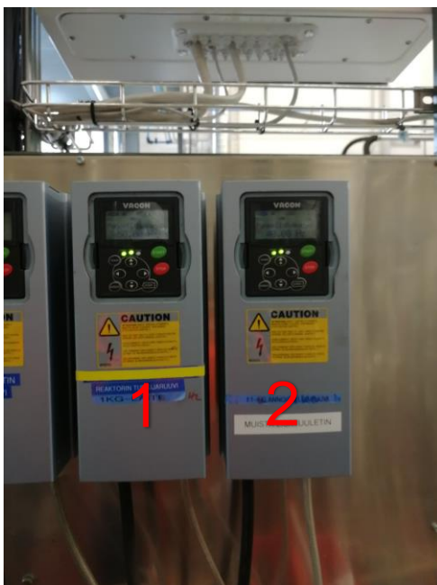
Image 4. Panel for the feeding- and pushing screw, 1: Screw conveyer frequency 2: Feeding screw frequency.
