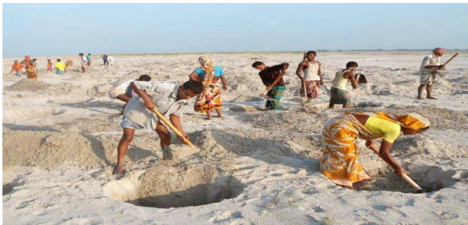
Figure 20. Digging process (practicalaction.org, n.d.)
