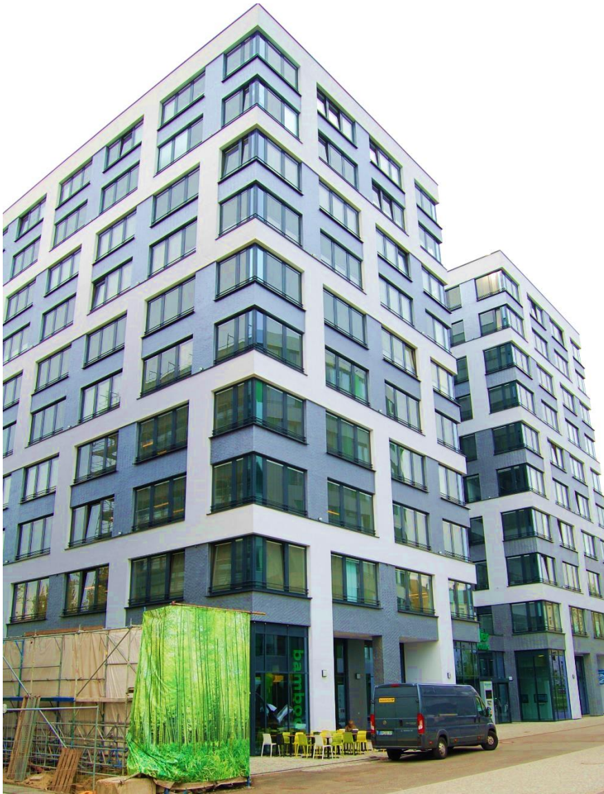
Fig. 19 Haus 12-13 View from the access road
