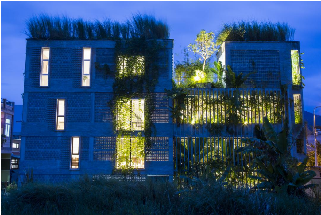
Figure 24. Southeast and southwest facades in the evening of the Alpes building
