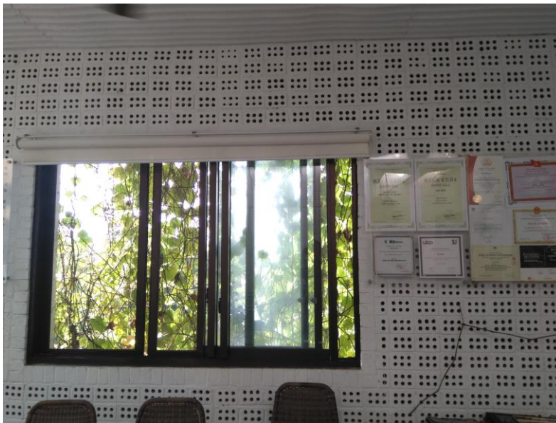
Figure 11. Hollow bricks were creatively placed for passive cooling
