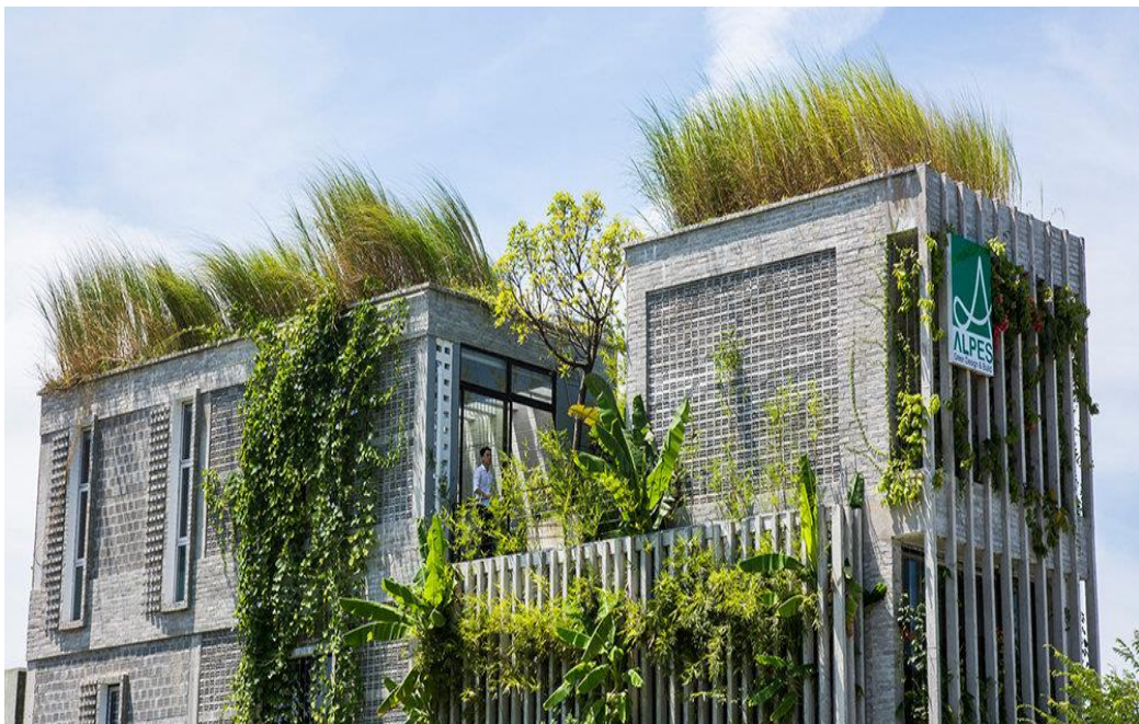
Figure 25. Green roof of the Alpes building
