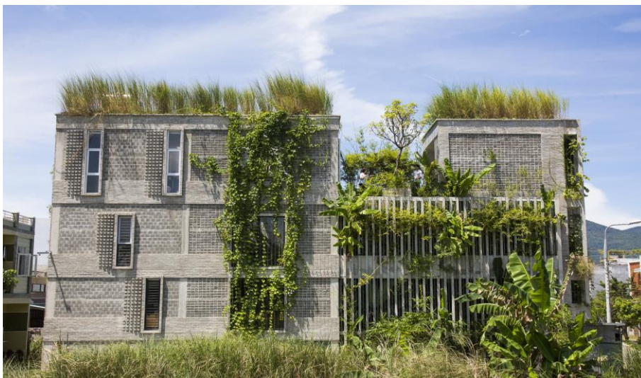
Figure 7. Southwest façade of the building [47.]
