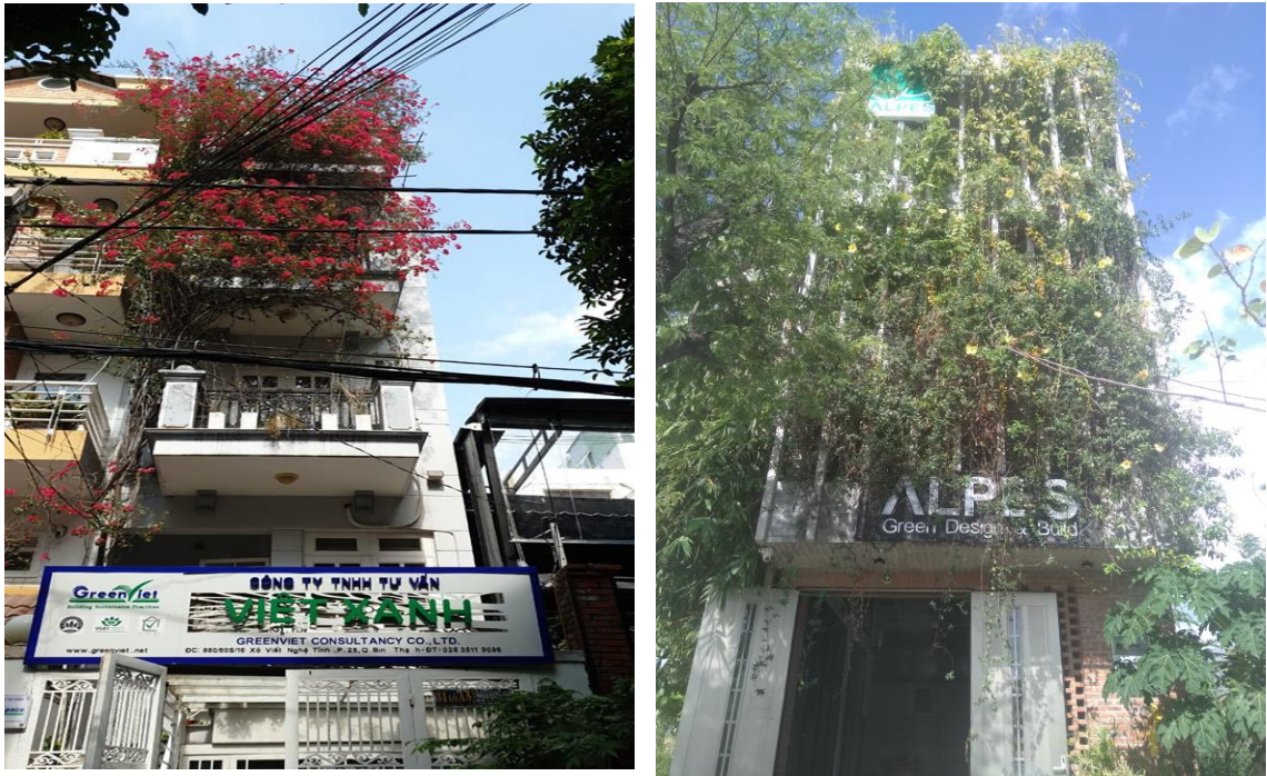
Figure 2. Front façade of GreenViet (left) and ALPES building (right)
