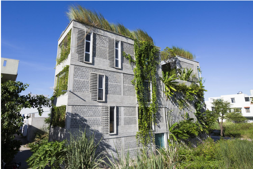
Figure 22. Northwest and southwest façades of the Alpes building
