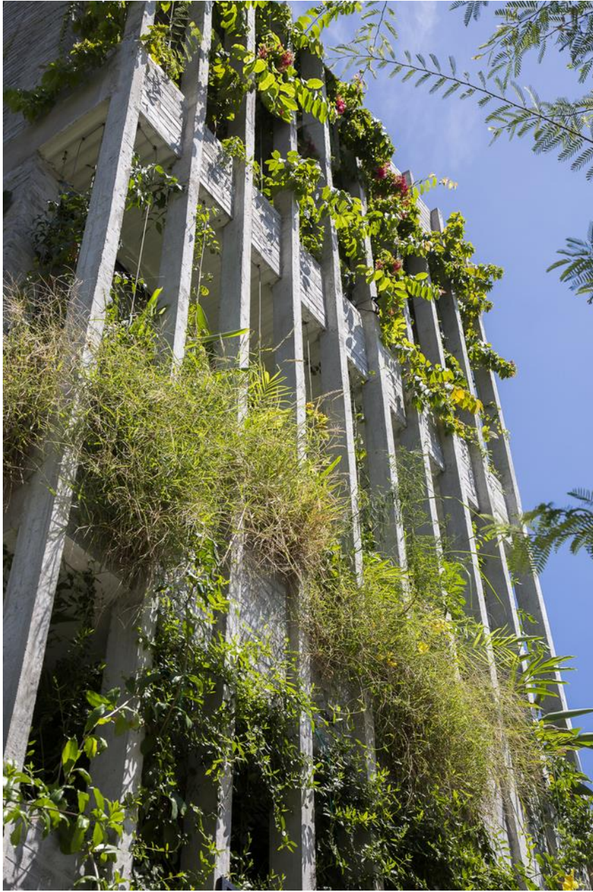
Figure 21. Southeast façade (with vertical sunshades) of the Alpes building
