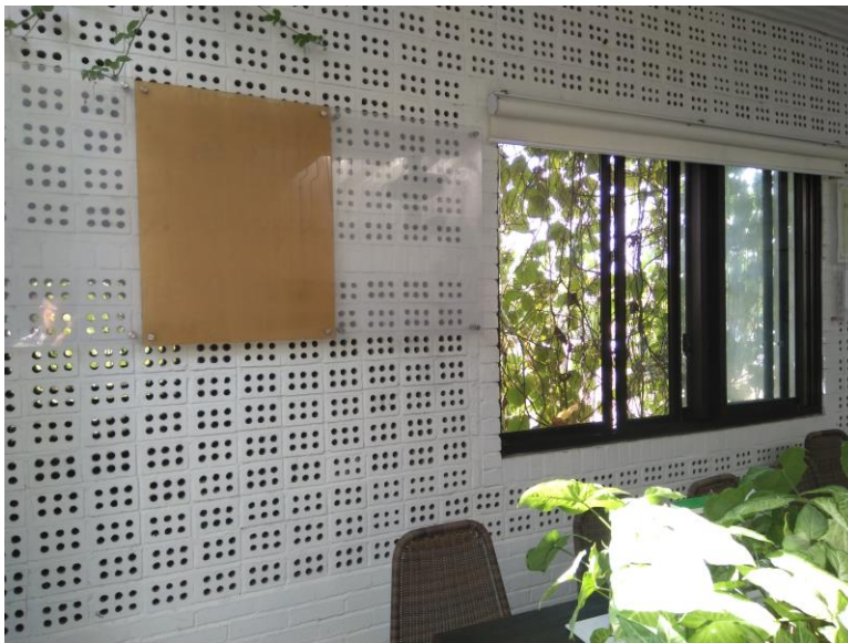
Figure 10. Brick holes create natural ventilation for the Alpes building
