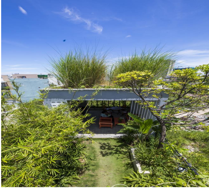
Figure 6. Green roof of the Alpes building [47.]
