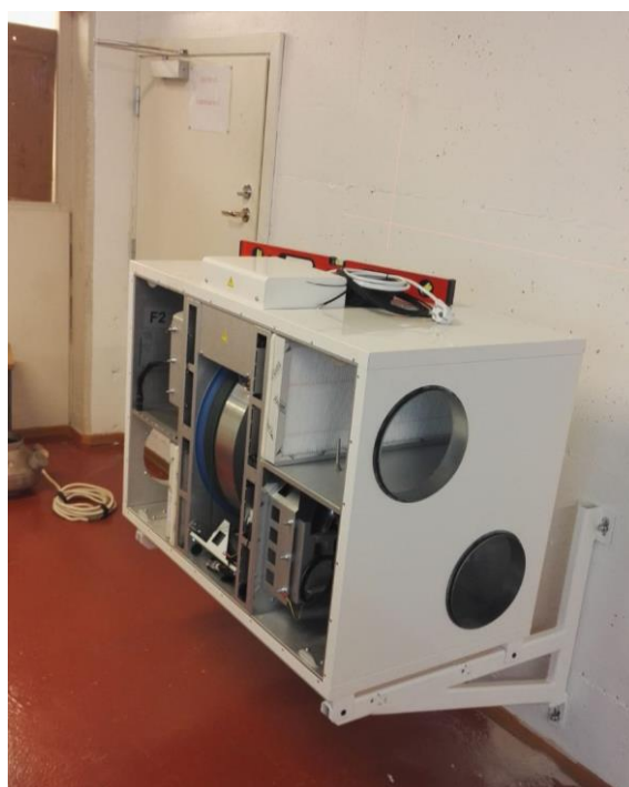
Figur 23. Ventilationsaggregat under installation
