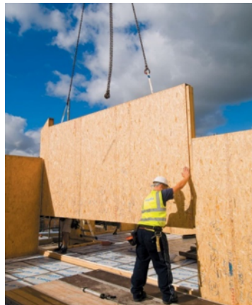
Figure 4. Massive timber element installation (Riley, n.d)
