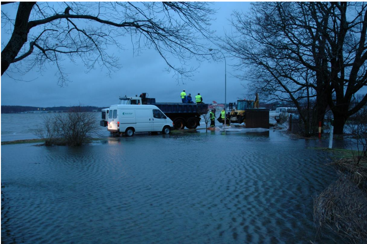
Figure 12: January 9, 2005 flooding in Ekenäs Old Town. Workers are attending to the power distribution box near Västvallen Road that failed. Photo by Sebastian Lindberg.
