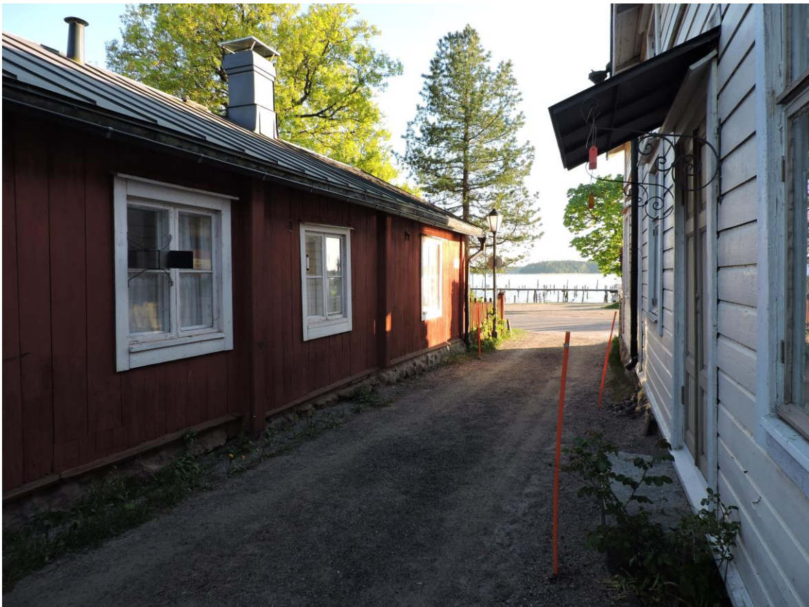
Figure 19: The Adolfsson House at Linvävaregatan 1. The house has a very low foundation which may be exceeded by coastal flooding in the future. Photo by © Jack Räisänen.
