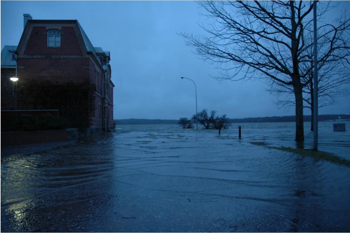
Figure 14: January 2005 flooding brought water over Västvallen Road. In this photo by Sebastian Lindberg, taken on January 9, 2005 at 9:12 am, water is seen reaching the steps of the Old Sauna.
