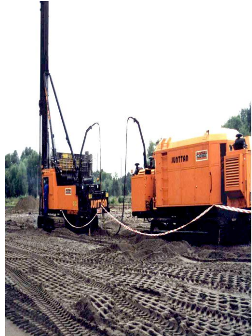
Figure 3.4.1b Deep dry mixing plant with separate binder silos, air drier and compressor
