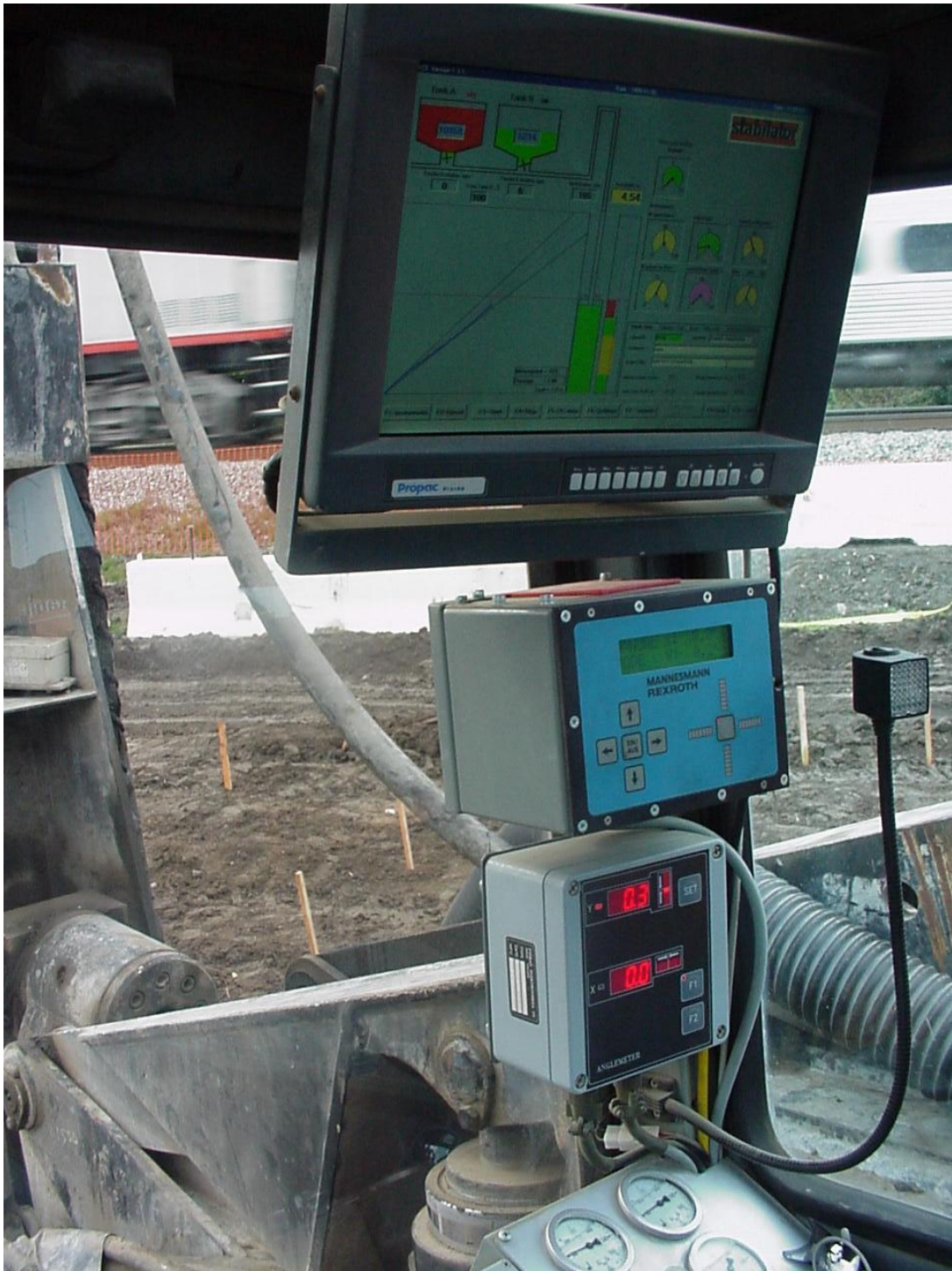
Figure 1 The display units as fitted in the operators cabin on the installation equipment
