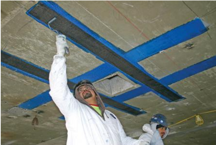
Figure 6.6 Strengthening the hole in the slab
