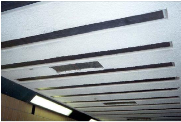
Figure 6.8 Laminates glued into the grooves (Teke brochure “Structure strengthening with composites”)
