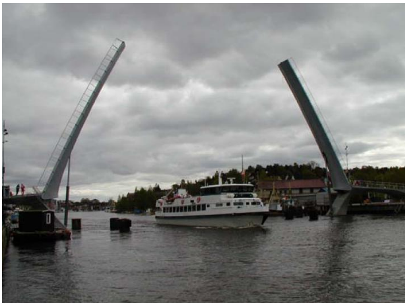
Figure 5.3 Opening footbridge in Fredrikstad, Norway
