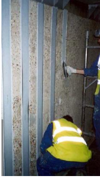
Figure 6.7 Strengthening of vertical structure (Teke brochure “Structure strengthening with composites”)
