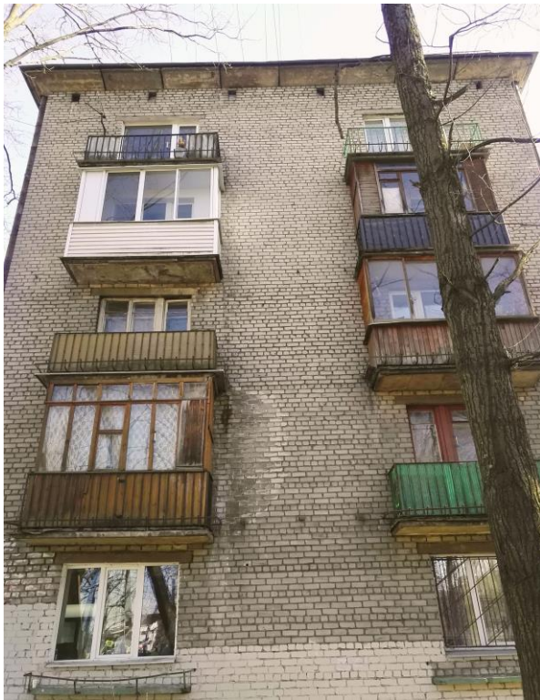
Figure 16. Detail of the external wall façade of the building at Lensoveta,83.
