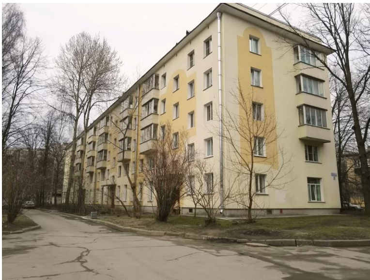
Figure 10. Renovation of building of series 1-528.
