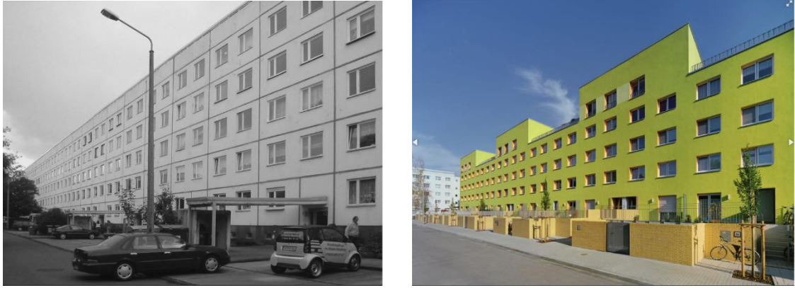
Figure 4. Paneled typical building before (left) and after reconstruction (right) [52].
