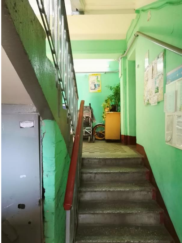
Figure 17. One of the common stairwells of the building at Lensoveta,83.
