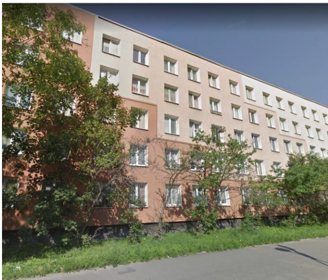
Figure 9. Renovation of building of series GI [66].
