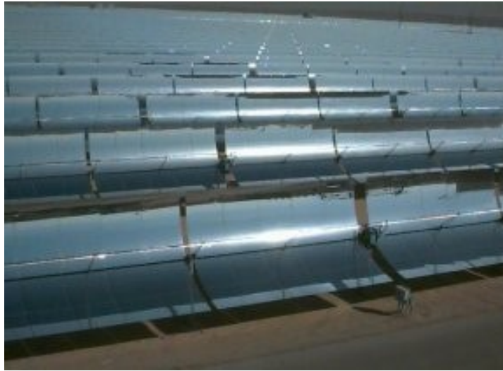
Figure 22. A power plant of parabolic solar collectors located in the Mojave Desert in California (Solar Thermal Power Plants , 2019)
