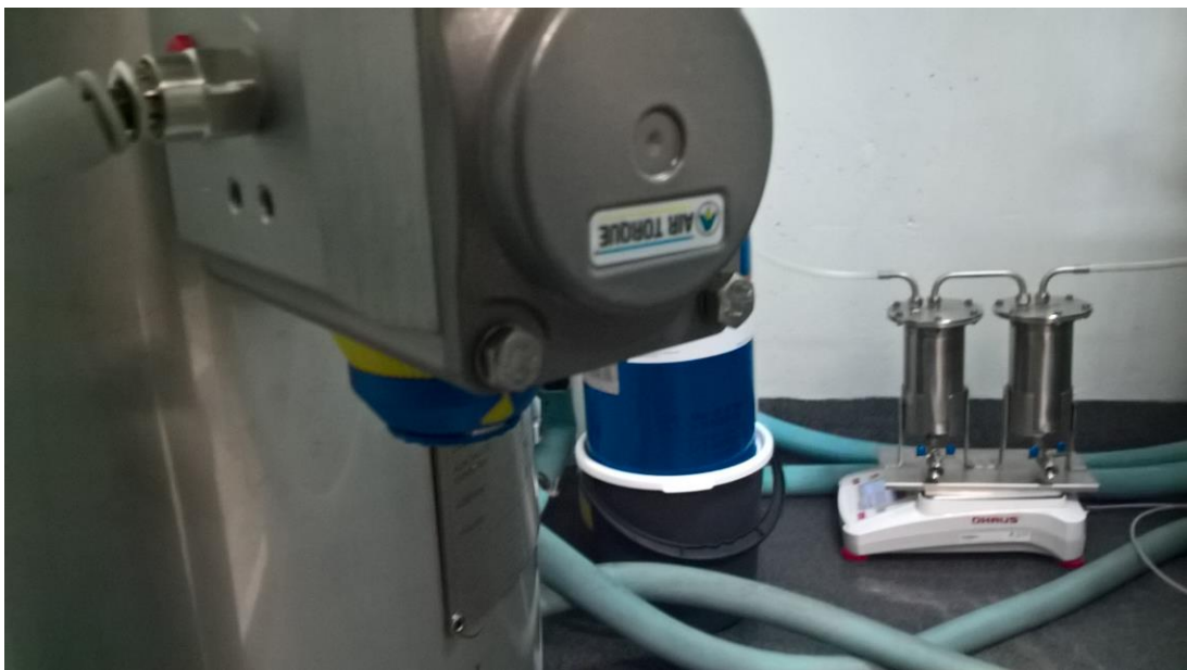
Picture 29. The automated valve SG1 in the opened position.
