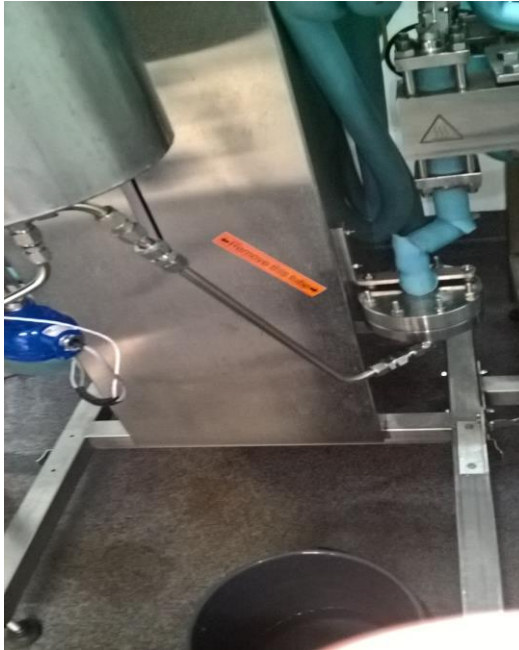
Picture 19. The tank prior to disconnecting the circulation pipe.
