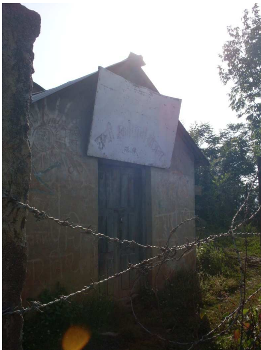
PICTURE 15 Ward 1 Reservoir Tank [36]
