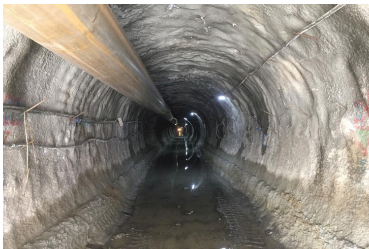
Figure 14: Tunnel Machinery (Shpati Gjollëshi. Gener2)
