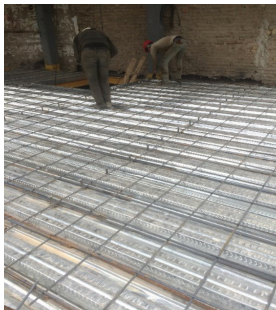
Figure 6: Steel deck Slab (Ehsan Bodaghi)
