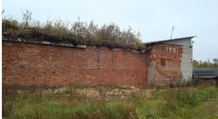
PICTURE 2. The technical conditions of constructions on the site.
