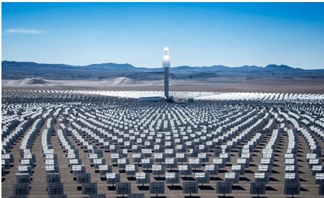
Picture 11. Concentrating solar power plant (Bureau of land management 2015.)
