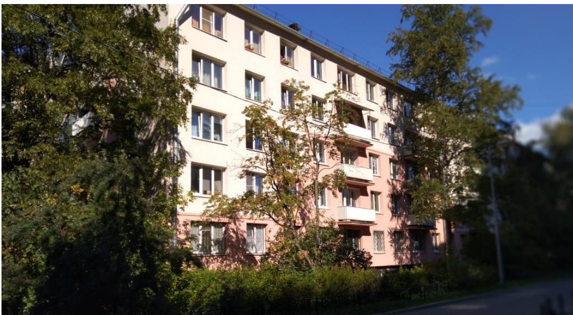
Figure 2.3. Renovated panel house. (Photo by the author)
