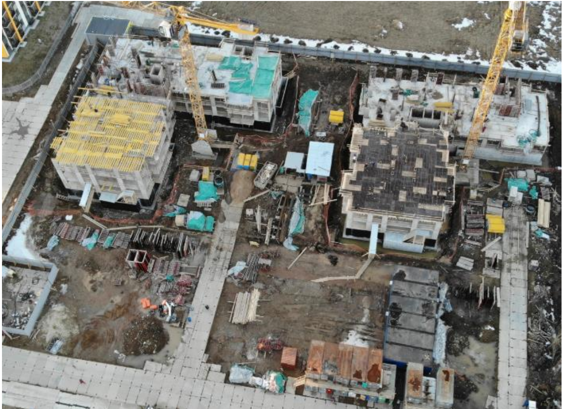
Figure 4.2. The view on the construction site in the city Pushkin. Photo was captured by a drone.
