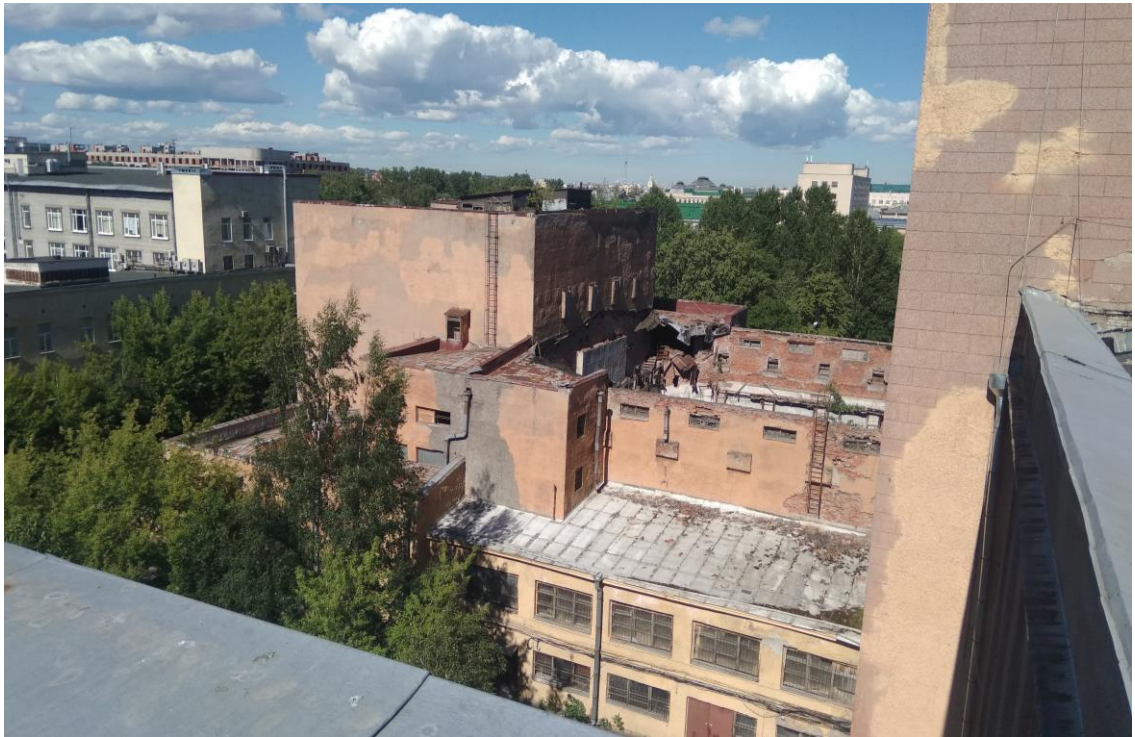
Figure 3.4. The Kirov's Palace of Culture in Saint-Petersburg. South wing. Collapse of the roof. (Photo by the author)
