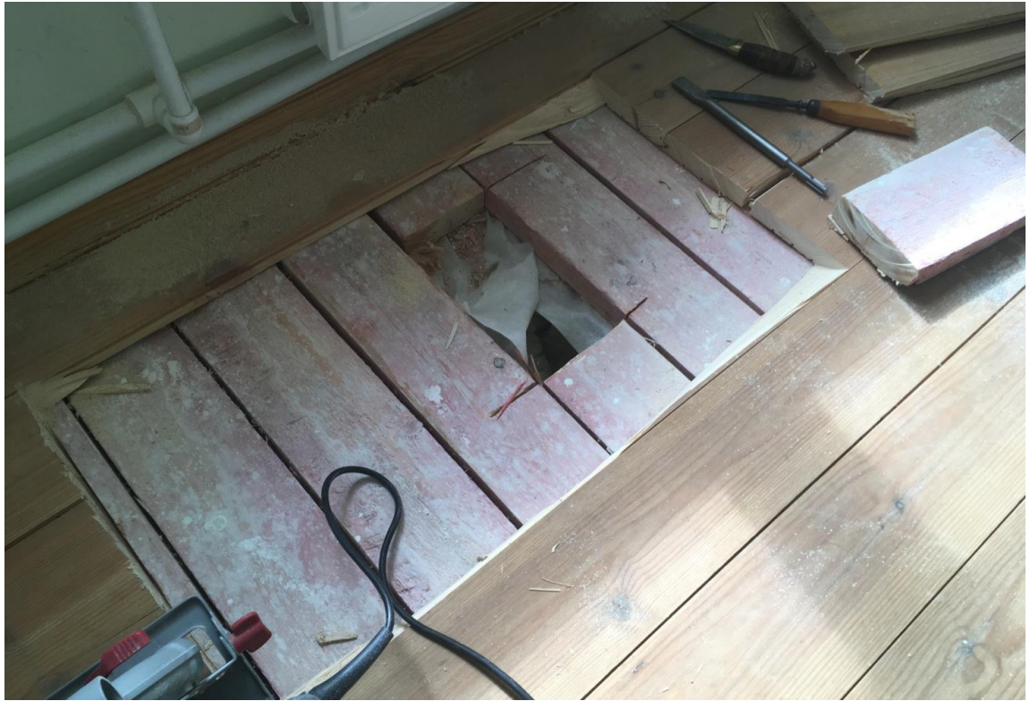
Figure 3.6. Sawed sector of the floor. (Photo by the author)
