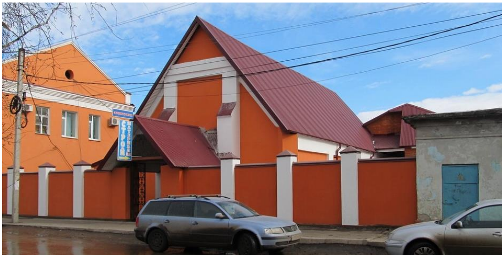
Figure 3.2. Jeiletz Deutsche Kirche (Currentry – building material shop) after inappropriate restoration. Lipetsk region. http://vif-vrn.ru/viewtopic.php?t=868
