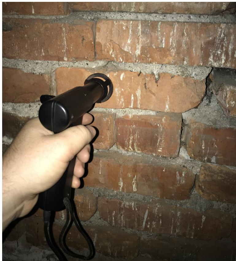
Figure 4.3. Using of the ultrasonic strength measuring instrument in Kirov's Palace of Culture. (Photo by the author)
