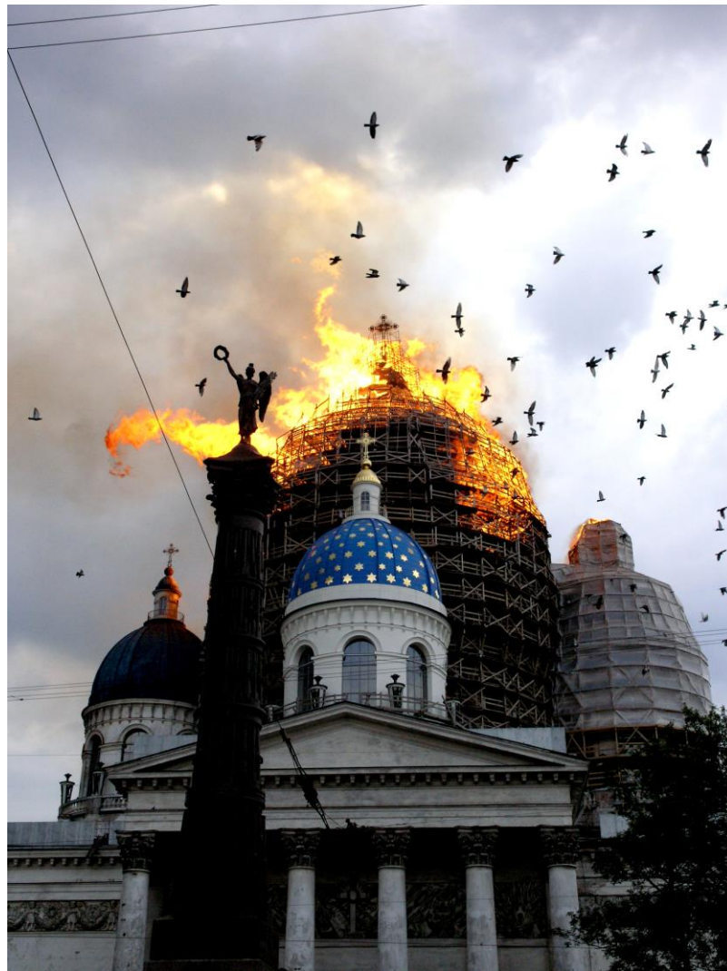
Figure 3.8. Fire hazard in The Cathedral of the Saint Life-giving Trinity. By Oleg Siromyatnikov - Praca własna, CC BY-SA 3.0,
