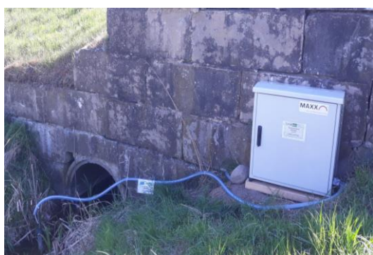
PICTURE 3. Installed automatic event sampler "Maxx" on site (Egliniski 2019)
