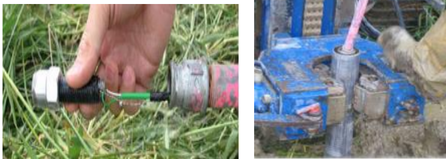
Figure 45. Installation of temperature sensor (Meinhard et al., 2014)
