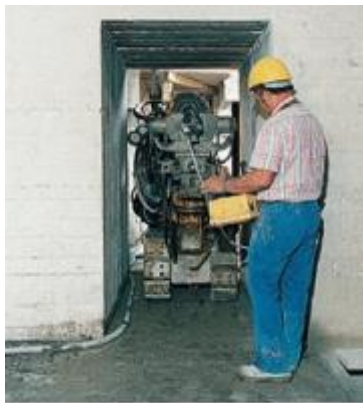
Figure 9. Jet grouting in confined space (Keller, 2017)
