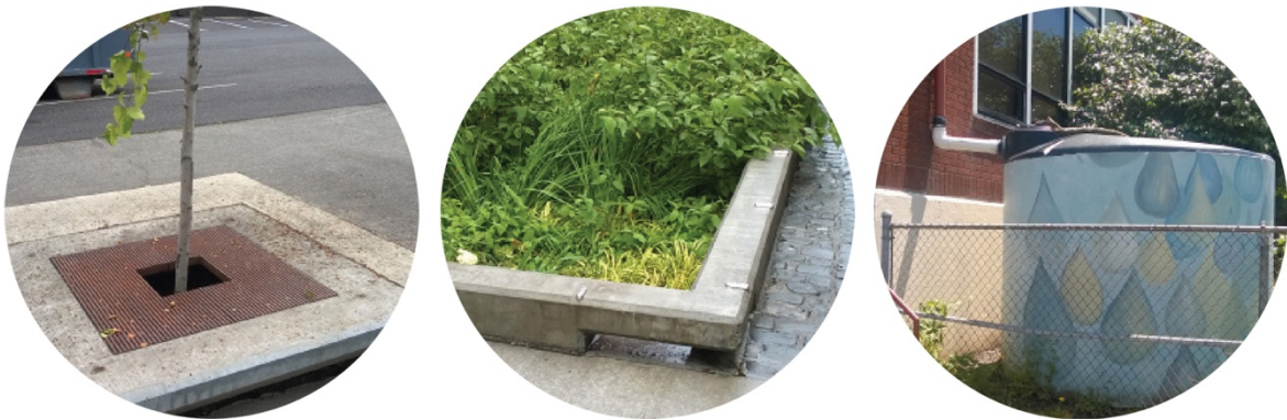
PICTURES 7, 8 and 9. Examples of a stormwater tree trench, stormwater planter and rainwater cistern. (Lähde & Ariluoma 2019.)
