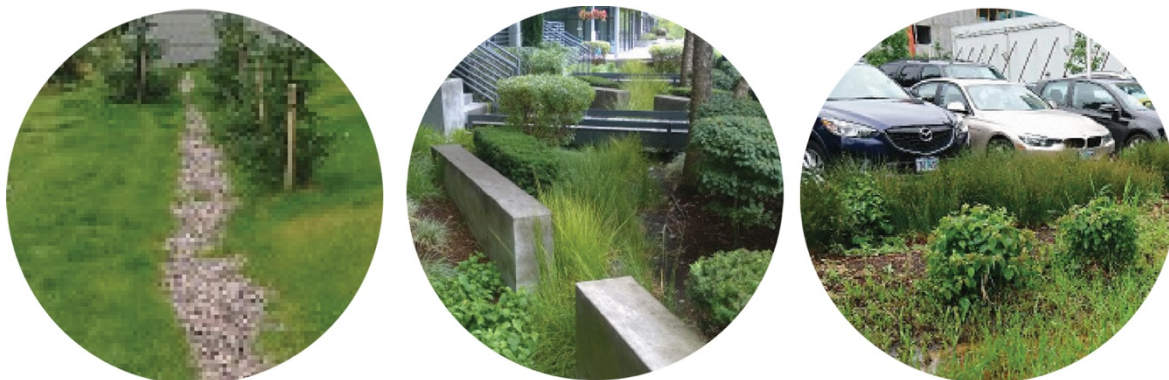
PICTURES 10, 11 and 12. Examples of an infiltration pit, rain garden and filter strip. (Lähde & Ariluoma 2019.)
