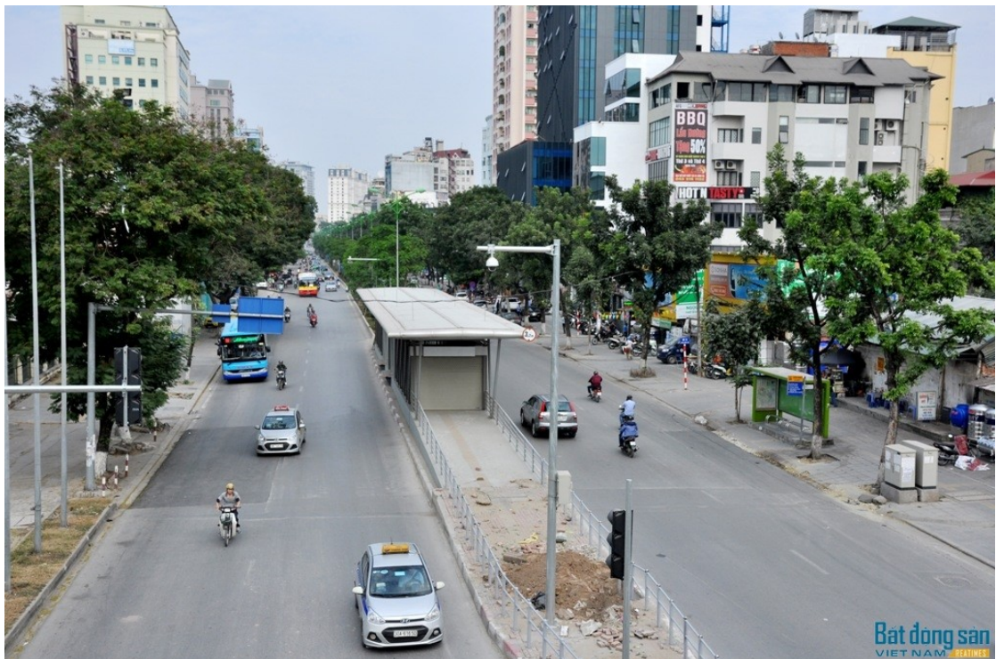
Unnecessary travel distance toward BRT stop from conventional bus stop.
