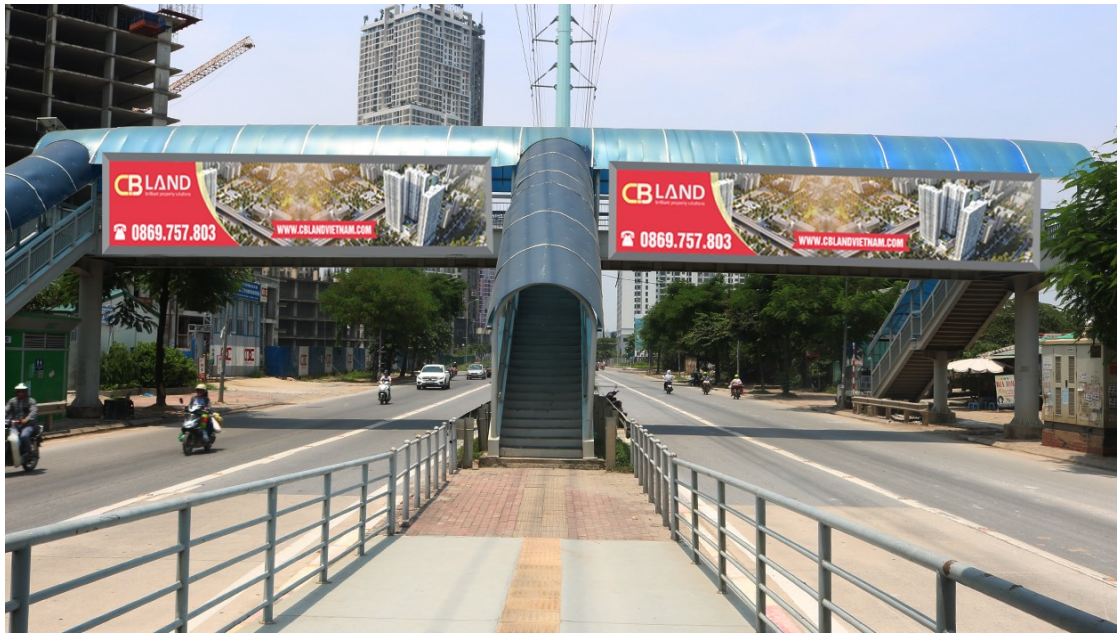
One sided overpass bridge.
